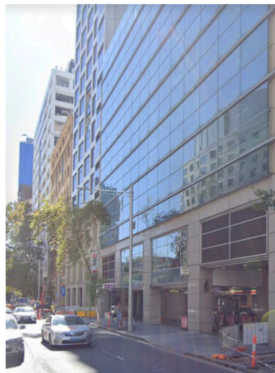
Photo of existing colonnade at Sussex Street
